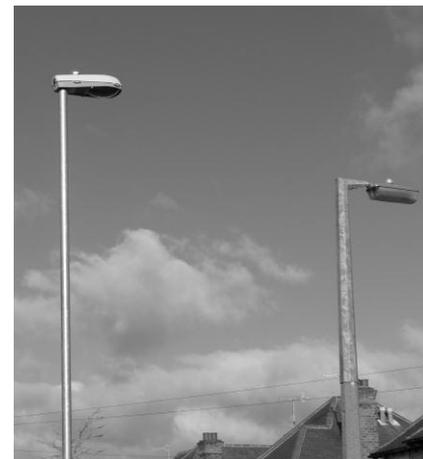
The columns are higher than the old ones to comply with modern standards. The design of lamps reduce upwards and backward spillage of light, they increase the light and spread on the pavement.
